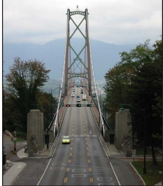
Reversible traffic lanes on the Lions Gate Bridge in Vancouver, BC, with overhead signals to indicate direction of traffic flow
